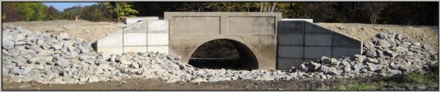
This 12-foot concrete arch bridge is one of three bridges on Depot Street that pass through the floodplain of the Contoocook River. It serves as a flood relief structure when the river overflows its banks. Constructed in 1914, it is considered historically significant and is eligible for listing on the National Historical Register.
