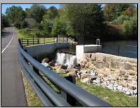
The Great Brook Cutler Shop Dam (NHDES Dam No. 009.12), constructed in 1925, consisted of a stone masonry spillway with concrete training walls and earth embankments at each abutment. The dam is influenced by the Summer Street Bridge located immediately downstream. The dam had deteriorated over time, had significant leakage, and was in need of repair.
